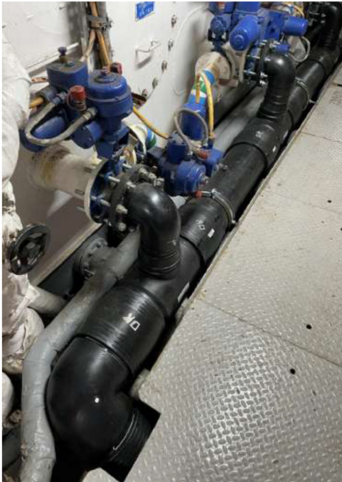
Suction and Feeding FW Manifolds
